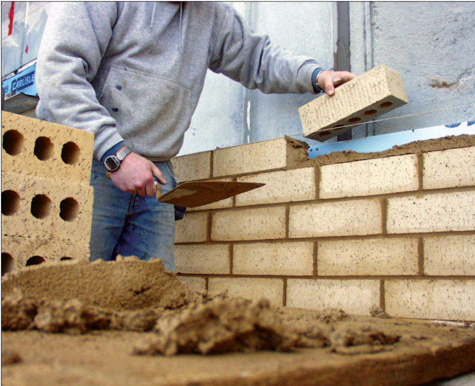
Consistent custom colored mortar, every time
