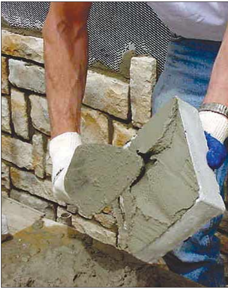
Stone Veneer Mortar is formulated for excellent workability.
