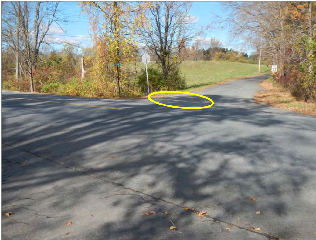
Figure 10. A second view of the Slate Quarry Rd/Wurtemberg Rd intersection looking north. Notice the faded stop line on Wurtemberg Rd (highlighted).
