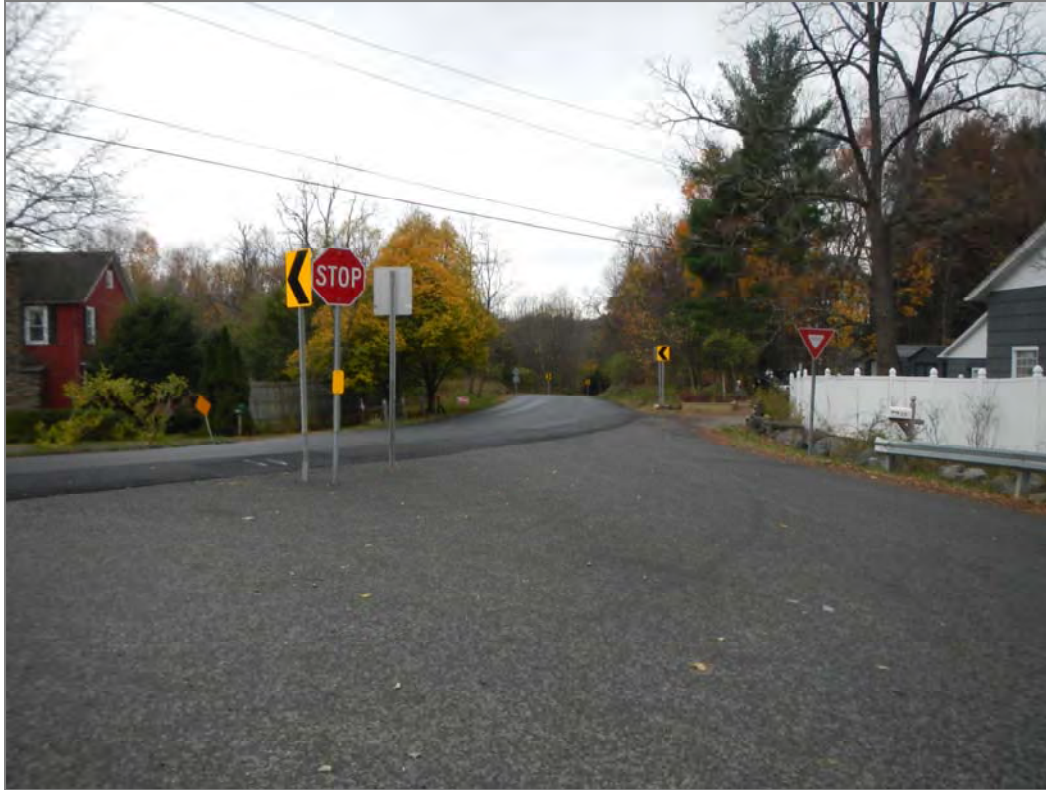
Figure 5. The intersection of Slate Quarry/White Schoolhouse Rd, looking west. The width of the intersection, coupled with the STOP and YIELD signs, creates a confusing situation for drivers.
