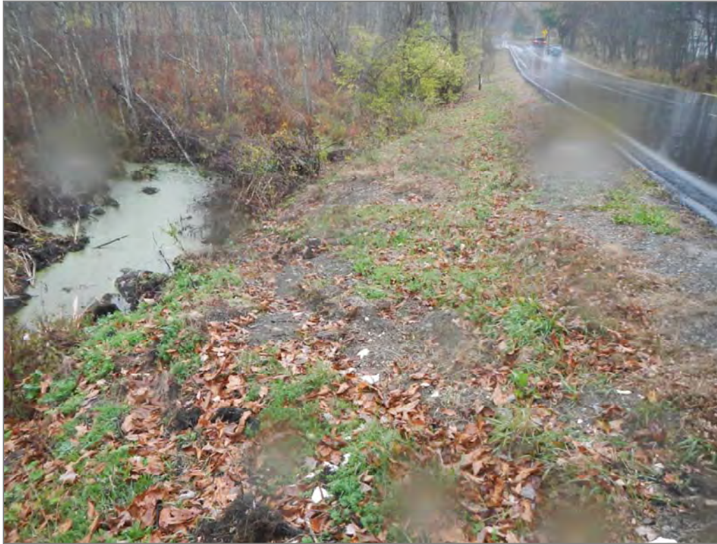
Figure 26. This area of Slate Quarry Rd may warrant guiderails to prevent vehicles from travelling into the adjacent swamp/marsh, as evidenced by the tire tracks in the shoulder.
