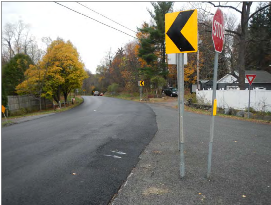
Figure 6. The width of the White Schoolhouse Rd approach to Slate Quarry Rd necessitates the placement of sign posts in the middle of the intersection.
