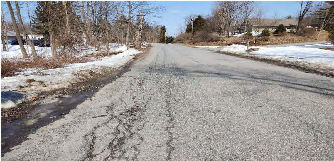
Example of Pavement not expected to last 5 years before major rehabilitation work is required.
