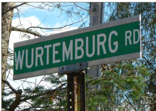
Figure 13. The street name signs in the study area (left) use the old lettering style that has now been superseded by a mixed-case style (above). Source: 2009 MUTCD.
