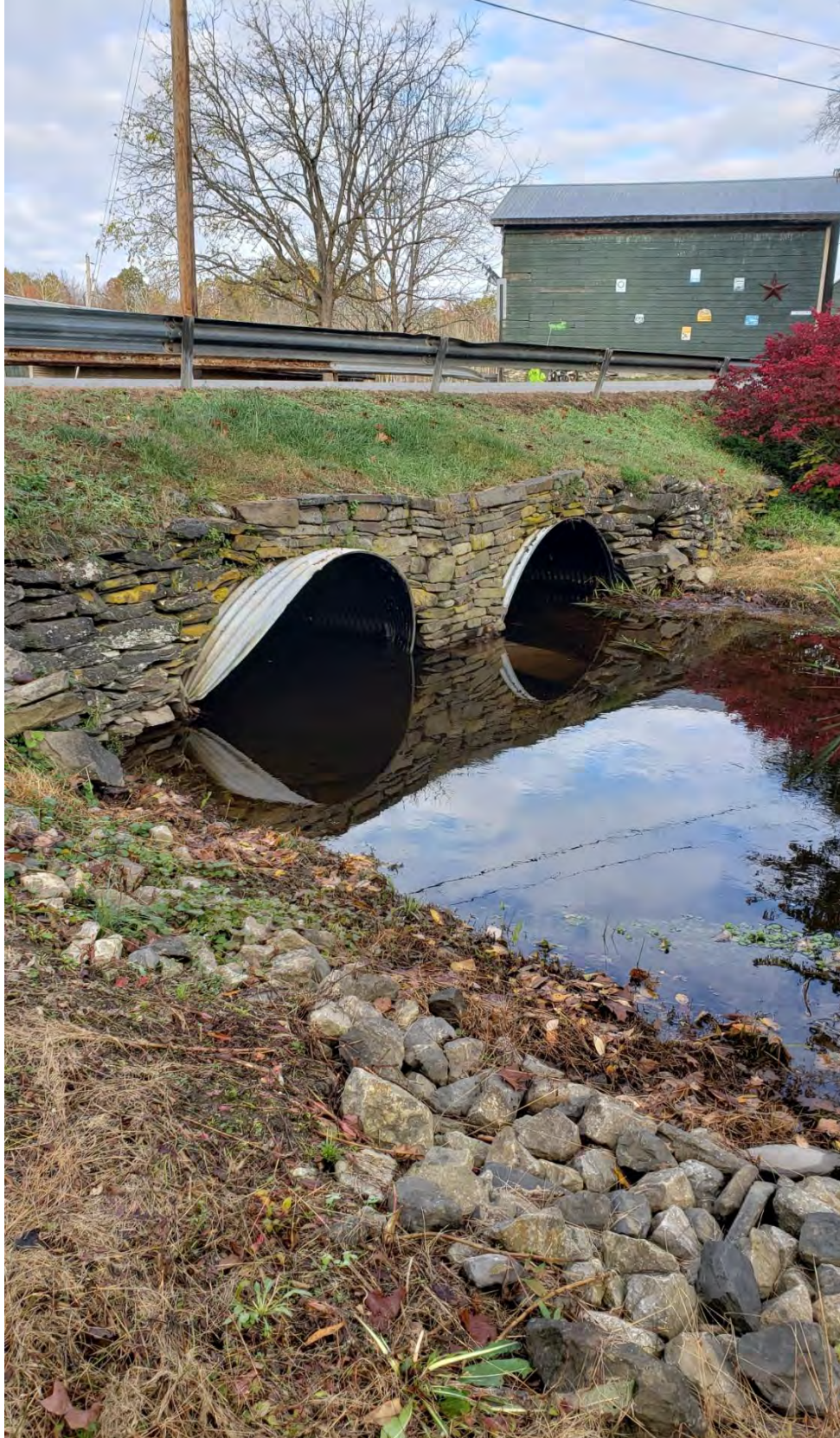
Deteriorating culvert and bridge
