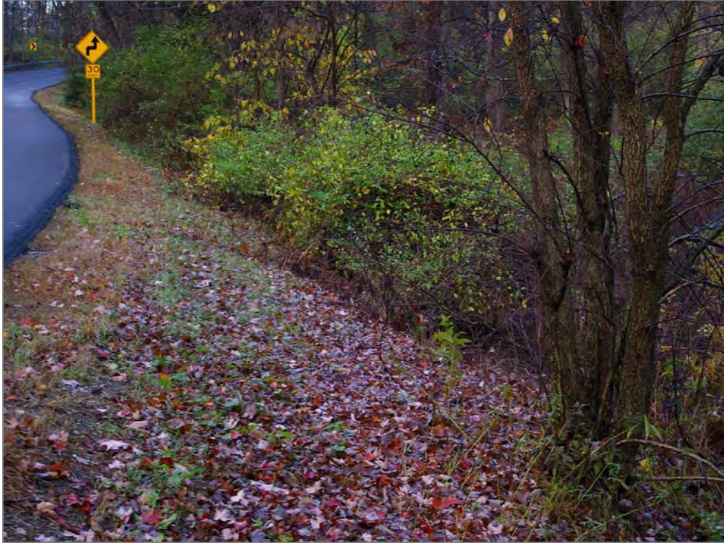
Figure 24. Sections of Slate Quarry Rd may warrant guiderails to prevent vehicles from travelling down steep embankments such as the one shown above.
