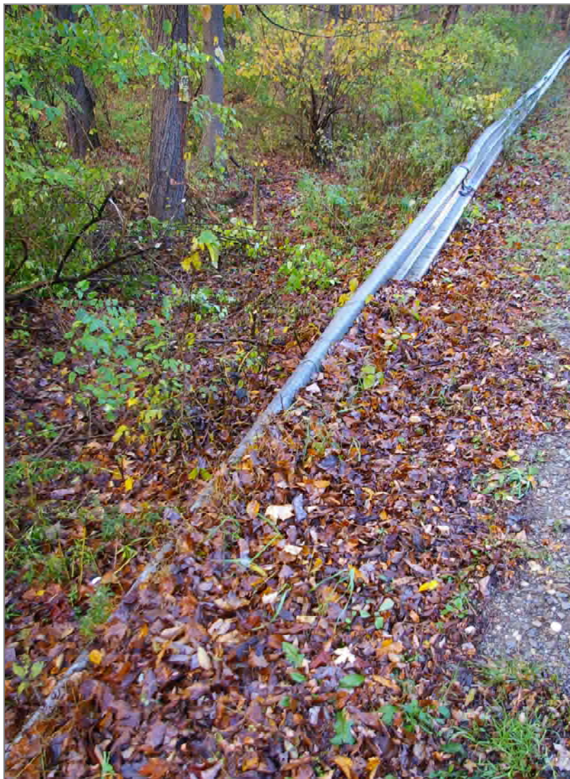
Figure 23. The guiderails along Slate Quarry Rd use the older “W-beam” design, which should be replaced with a “box-beam” design (as shown above on CR16 ). A significant issue with the “W-beam” design involves the end treatment, which can act as a ramp for vehicles that depart the road.
