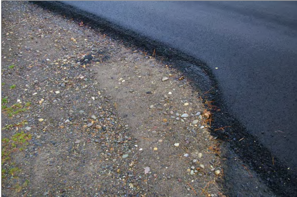
Figure 11. Due to the recent repaving, the shoulders along Slate Quarry Rd have steep drop-offs, which can destabilize errant vehicles.
