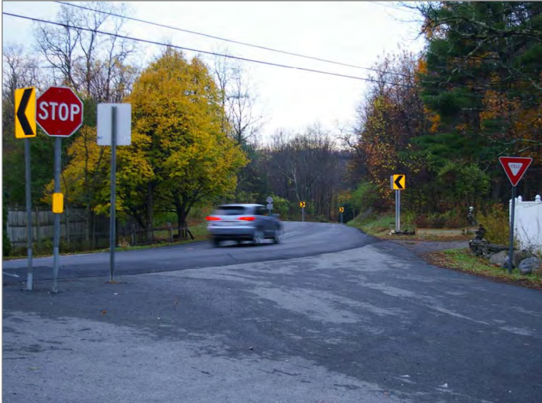
Figure 15. The Slate Quarry/White Schoolhouse Rd intersection looking west. Note the width of the intersection and contradictory STOP and YIELD signs.
