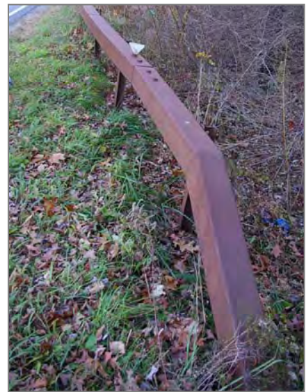
Figure 22. Some of the guiderails along Slate Quarry Rd are in need of repair (left), while delineators should be checked for retro-reflectivity (right).
