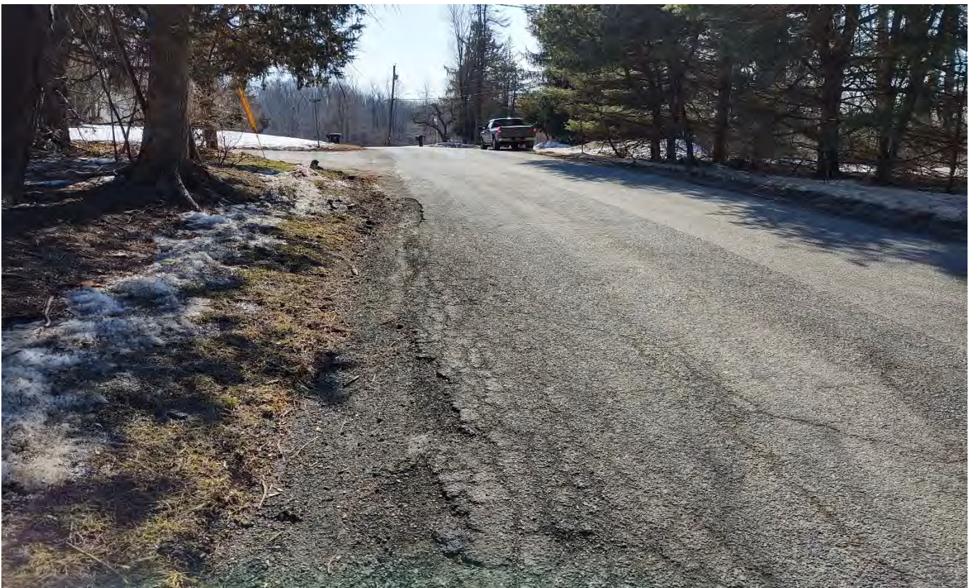
Photo above- Pavement edge and shoulder are breaking, typical condition in several areas.
