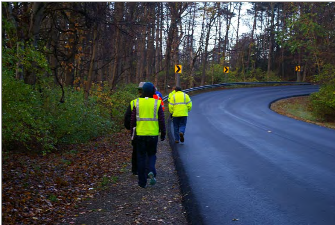
Figure 12. The steep pavement edges make it difficult to walk or bike along Slate Quarry Rd.
