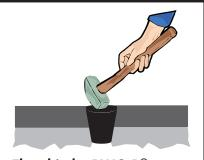
Then hit the PLUG-R® directly with the hammer to break off any excess asphalt. The PLUG-R® is now part of the pavement.
